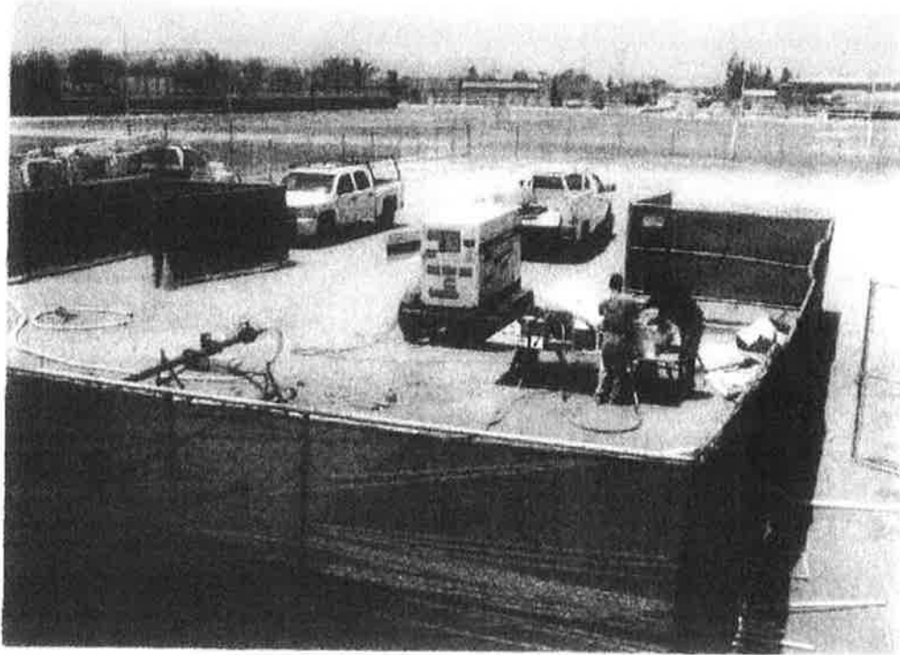
Parameter of water well construction site approximately 30'x30'
